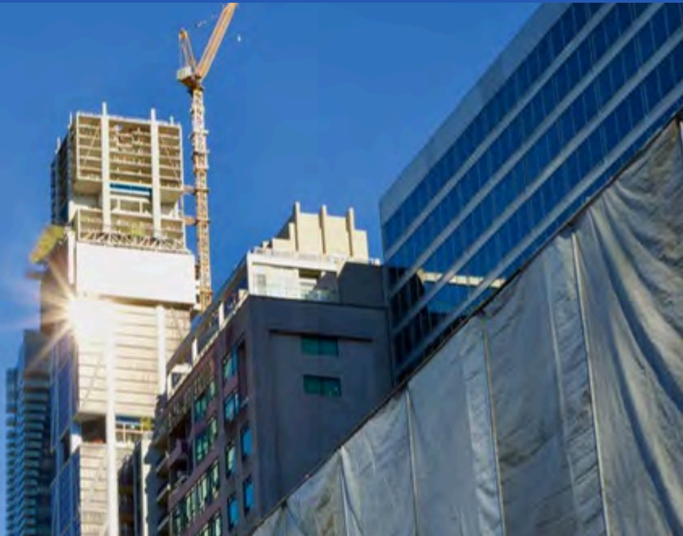
Ongoing construction at One Bloor West
